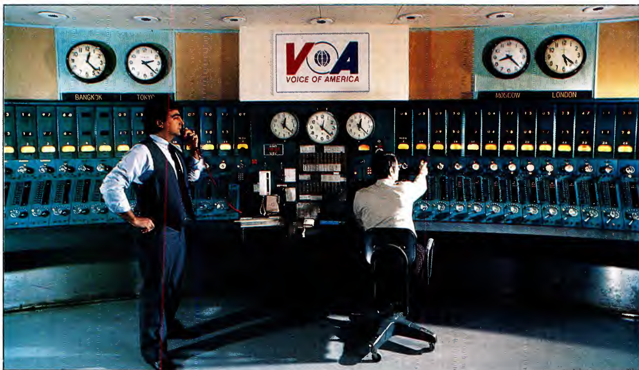
The old Voice of America master control room. Built in the early 1950s, the facility was used until recently to transmit programming in a wide variety of languages to the far-flung VOA system. The equipment shown was designed by Gates Radio to distribute 26 different programs simultaneously from 100 different sources. (Courtesy of VOA.)
